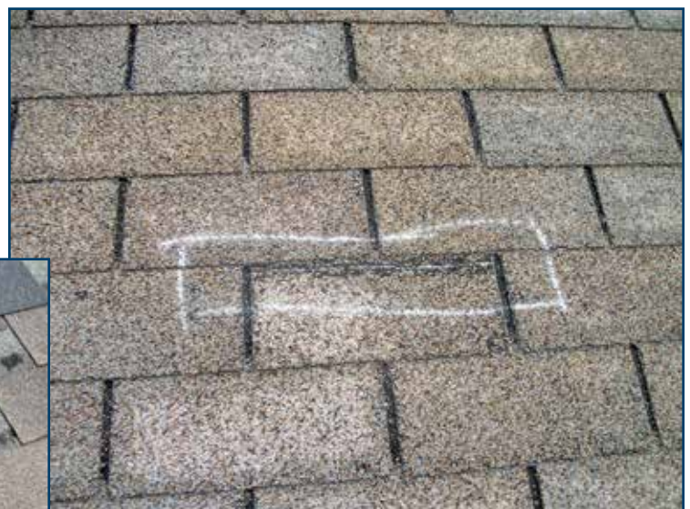
Figure 10 – Natural linear folding/creasing that constitutes legitimate roof damage. Note also the “graying-out” of the crease, suggesting this tab has been flexing in the wind for some time.
